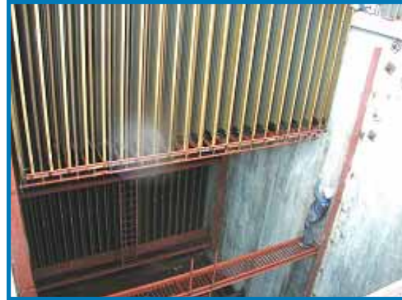
Placement of new field
