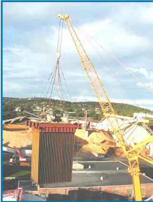
Lifting in new internals
