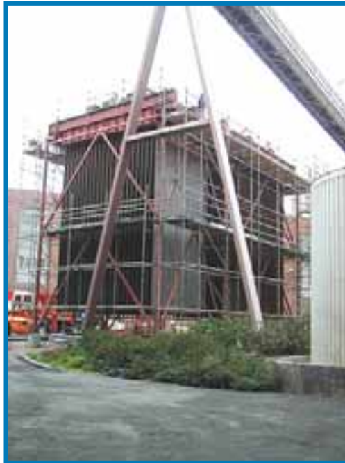
Erection of collecting plates in rack
