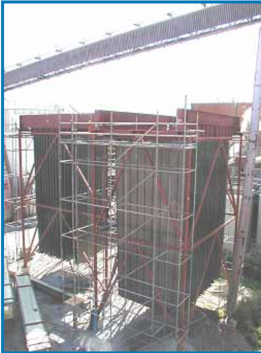
Erection of collecting plates in rack
