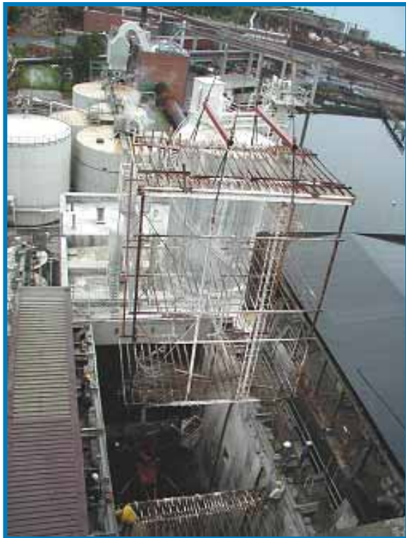
Removing of old internals
