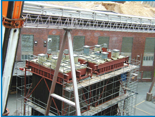
Erection of rapping gears in rack
