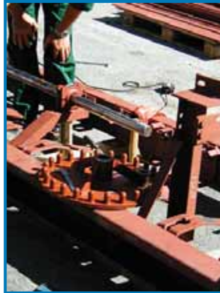
Pre-erection of rapping gear
