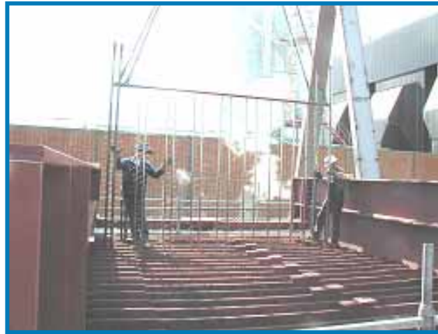
Erection of discharge frames in rack
