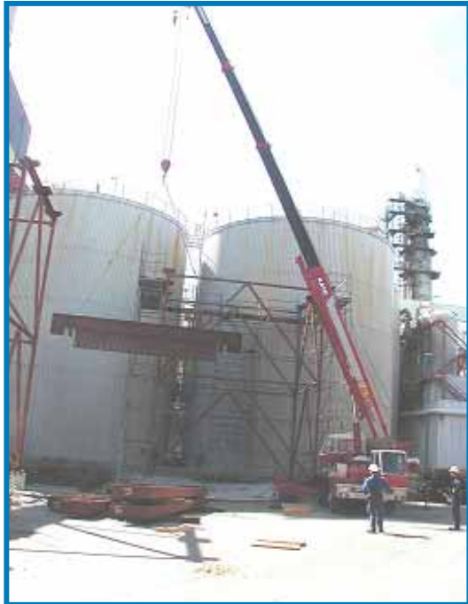
Top frame to be placed on rack
