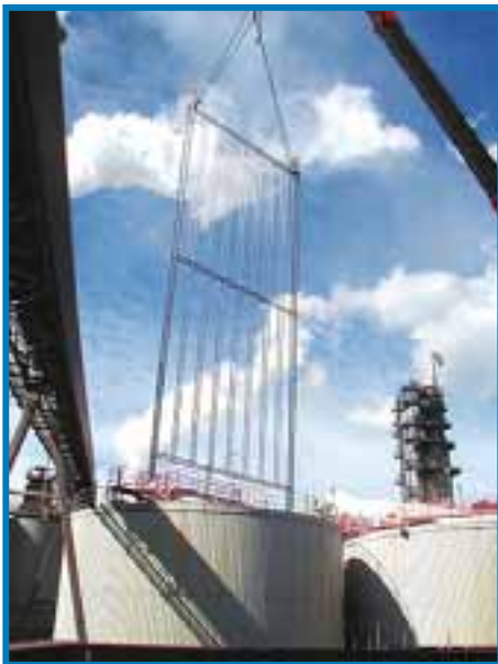
Erection of discharge frames in rack
