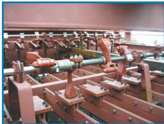
Erection of rapping gears in rack
